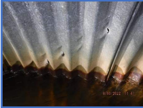
Image 7 – Three ½ Inch diameter holes at 107 feet
