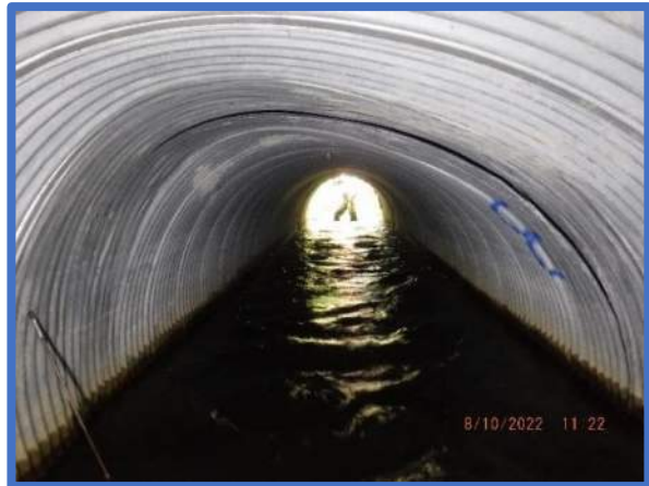
Image 4 – Deformation with 14% ovality at 33 feet
